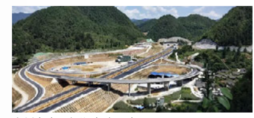
贵州乌当至长顺高速公路 Guizhou Wudang to Changshun Expressway
