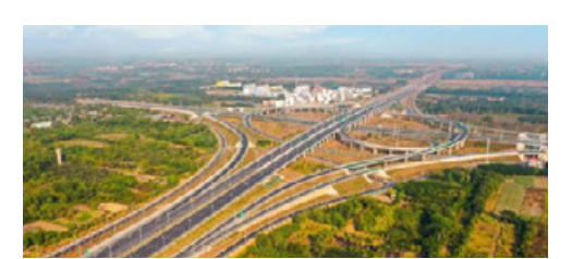
广西钦州至北海高速公路 Guangxi Qinzhou to Beihai Expressway
