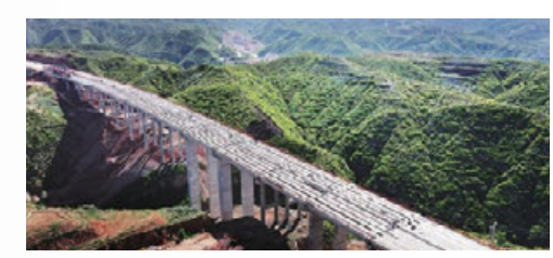
山西太原西北二环高速公路 Shanxi Taiyuan Northwest Second Ring Expressway
