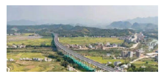
广东怀集至郁南高速公路 Guangdong Huaiji to Yunan Expressway
