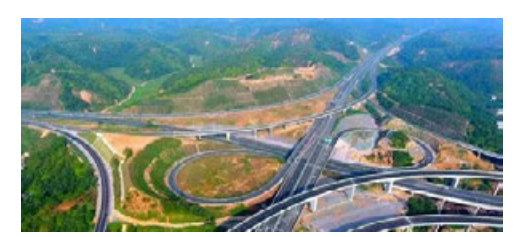
贵州都匀至香格里拉高速公路 Guizhou Duiyun to Shangri-La Expressway
