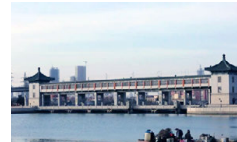
天津市海河口泵站 Tianjin Haihekou Pumping Station
