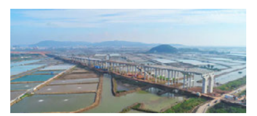
广东珠海鹤洲至高栏港高速公路 Guangdong Zhuhai Hezhou to Gaolangang Expressway
